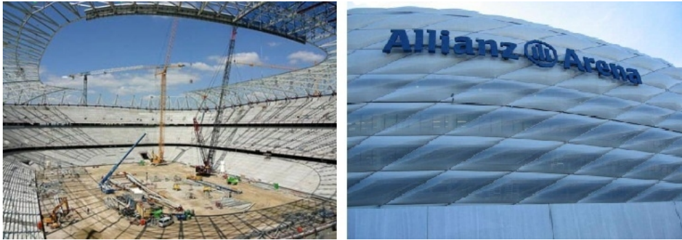
Picture 4. ETFE Diamond-shaped masses and established bases on steel structure covered with glass display at the Allianz Arena (6-8).
